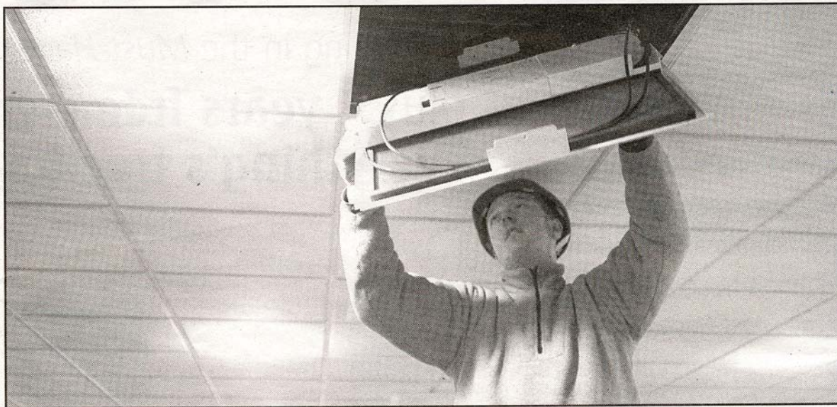
NEW PRODUCT : A workman fits an i-ceiling loudspeaker system
